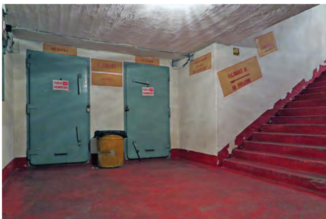
Inside shelter number 9. Most of the individual rooms within are now used as rehearsal space
